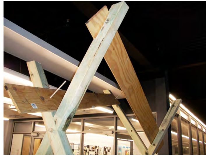
we added reinforcements to give us the needed cross bracing
