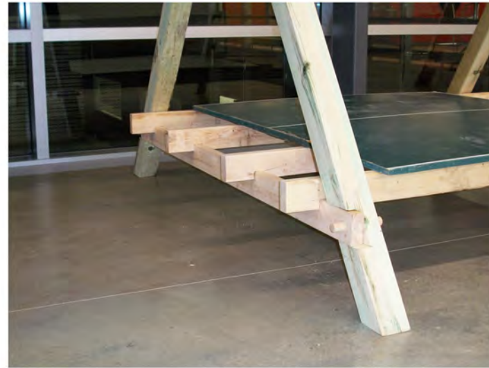
we used strong groved in connections to hold the base up
