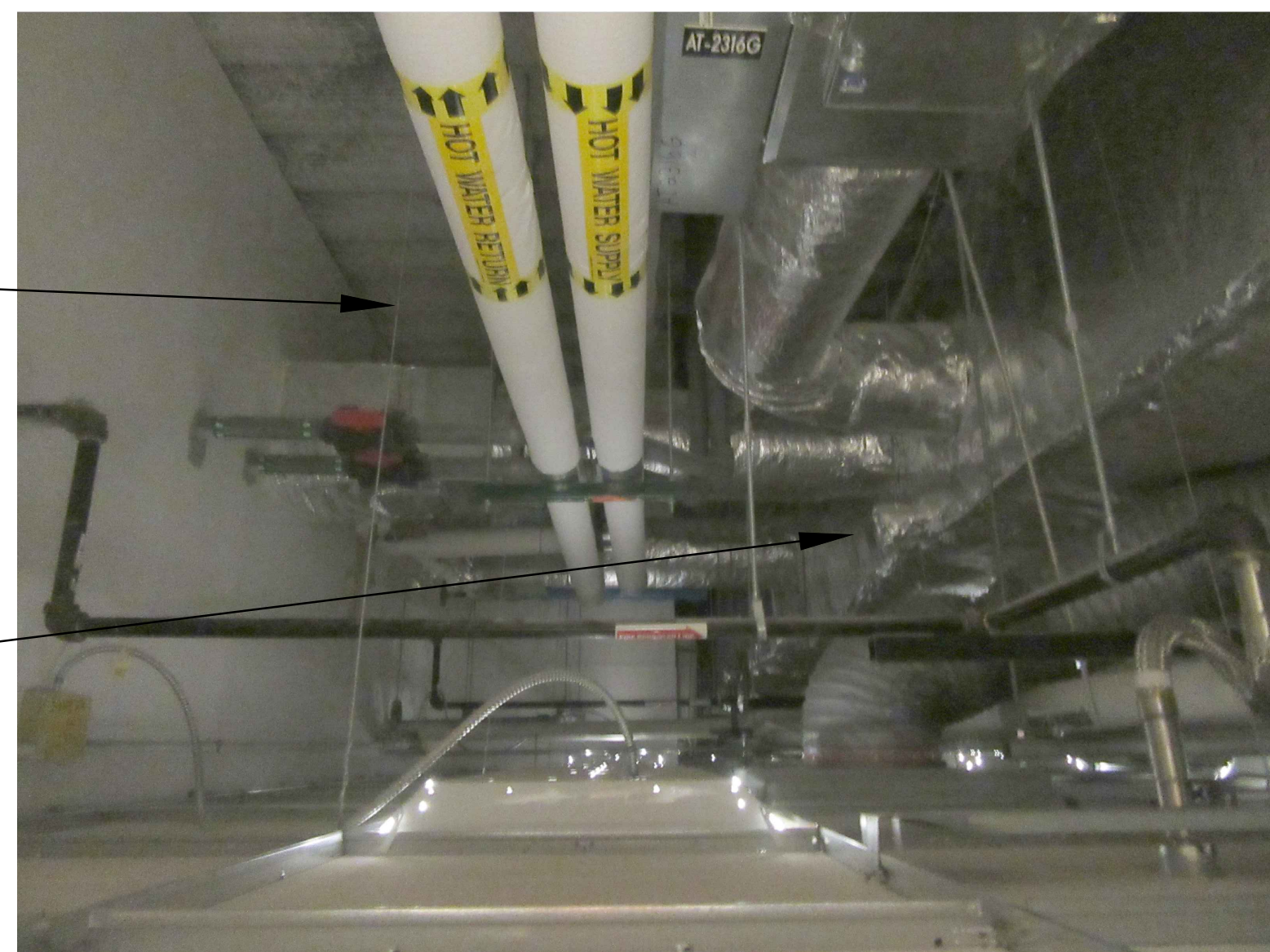
5 DUCT ROUTING - HALLWAY
