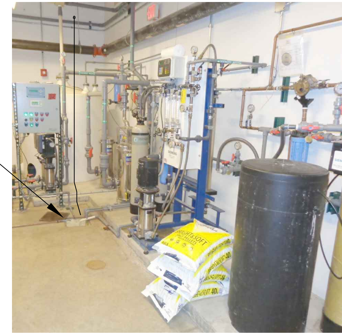
4 FLOOR DRAIN LOCATION - MECHANICAL ROOM
