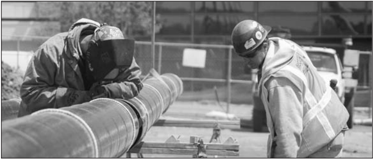
Construction continues on the HCNS site on Wednesday.
