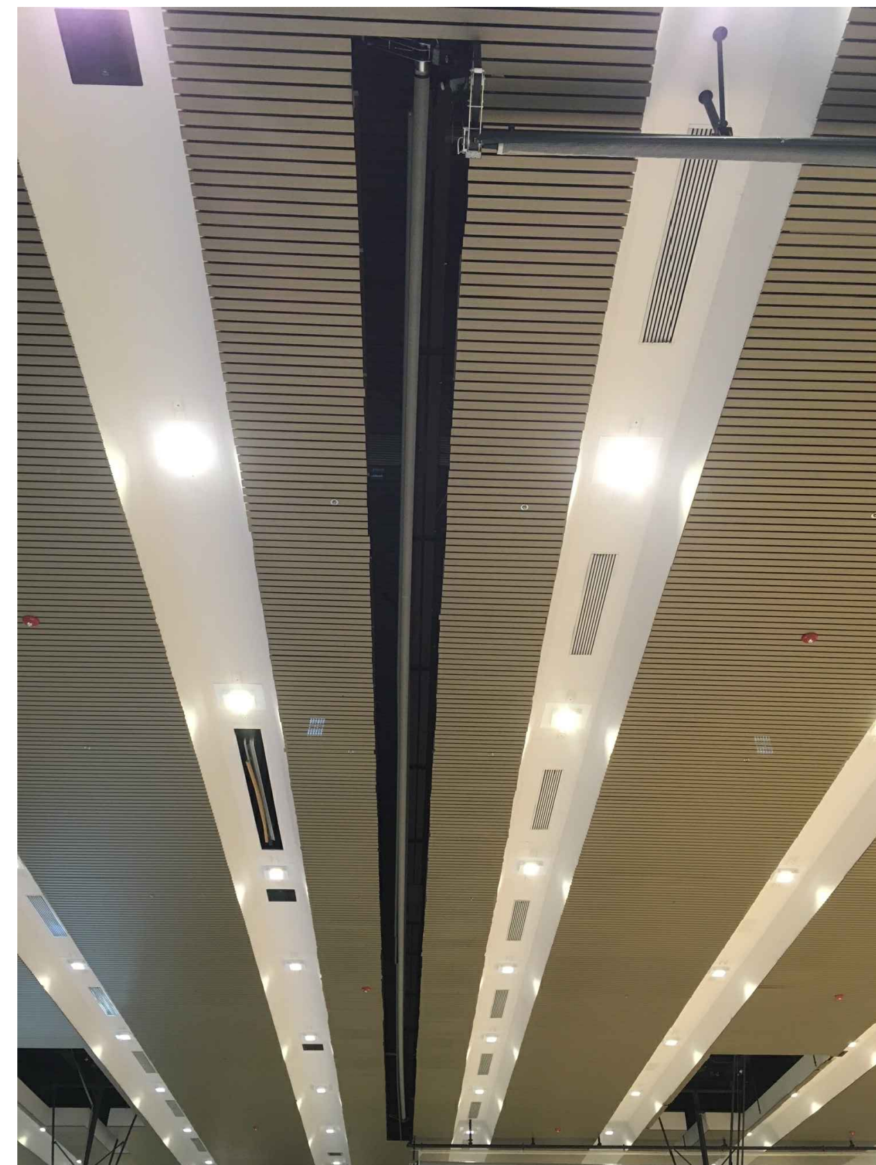
EXISTING RECESSED CURTAIN (NORTH/SOUTH)
